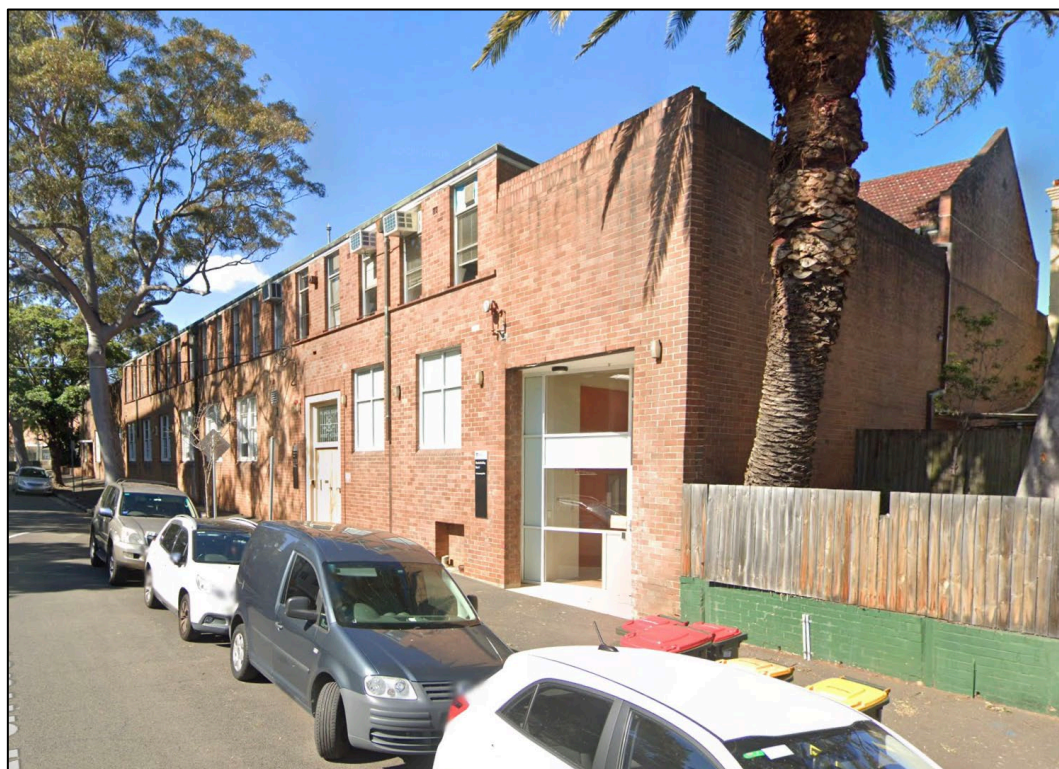
Mackie Building, 2 Arundel Street, looking east
