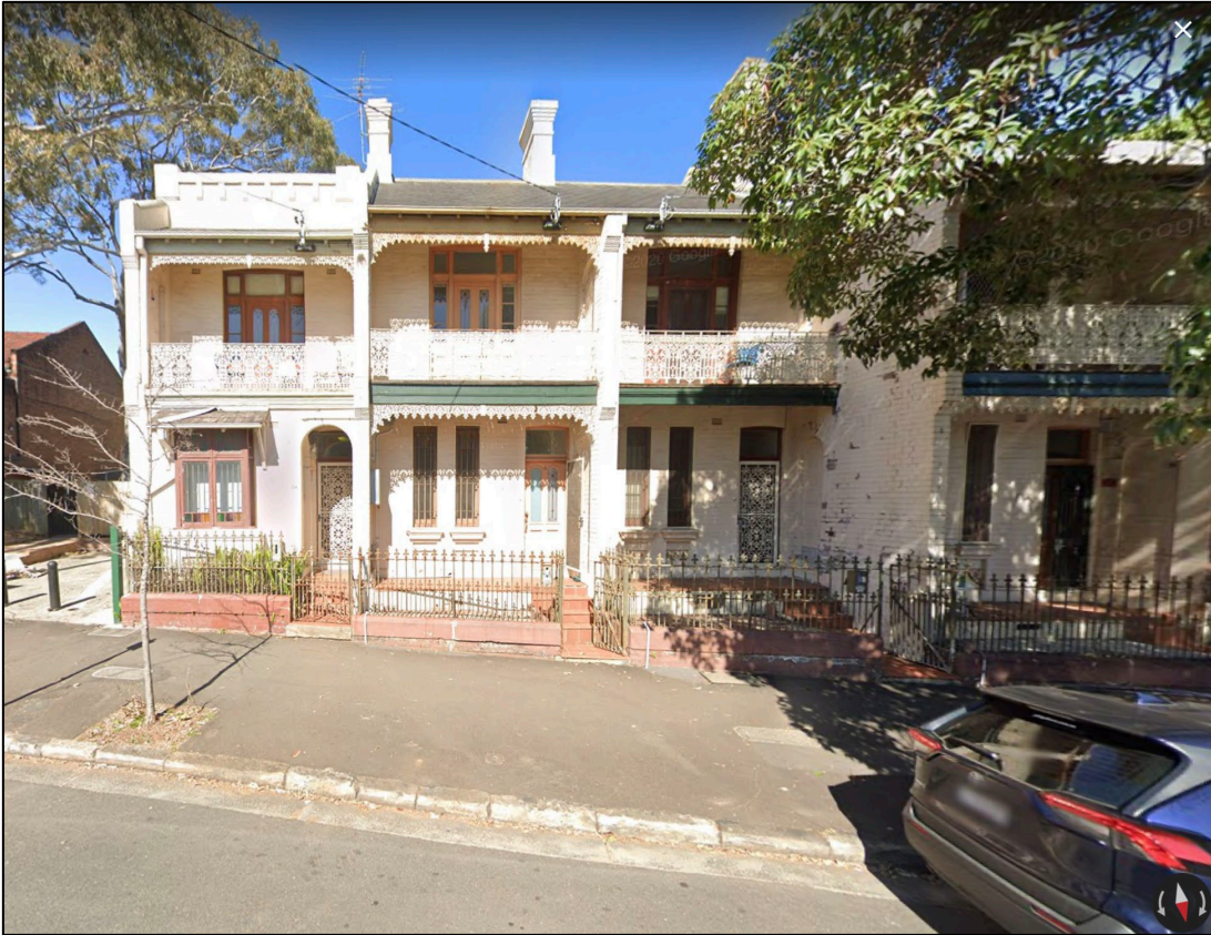
Terraces 2A, 4, 6 & 8 Arundel Street, Forest Lodge
